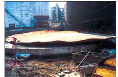
ABOVE: Collapsed sulfuric acid tank (photo from the Delaware-on-line News Journal). Smaller photo shows the uplifted floor due to the internal deflagration.
